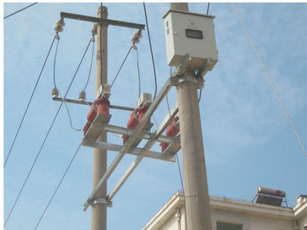
(f)户外-10kV馈线快速短路保护
