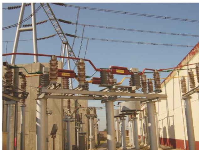
(i)户外-大容量变压器35kV侧快速短路保护 (硬母线桥安装)
